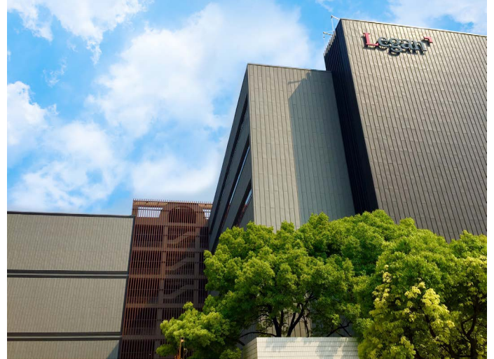
WaiGaoQiao Data Center
