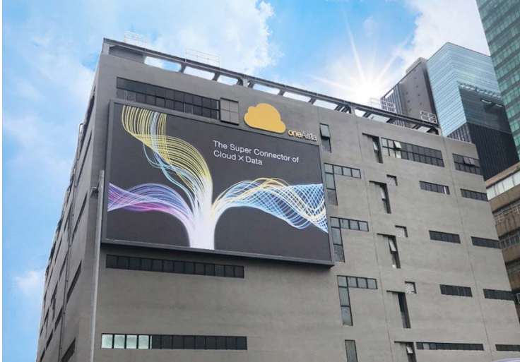
Kowloon Bay Data Center
