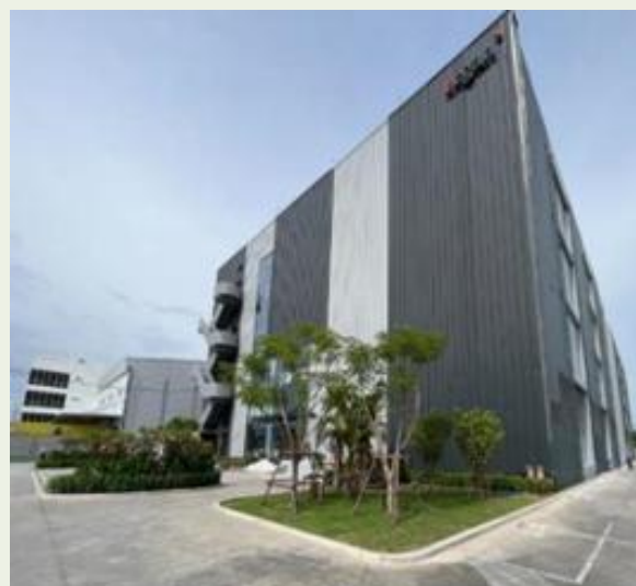
(Thailand – North Bangkok BKK1 Data Center)
