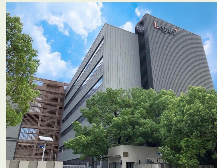
(Shanghai – WaiGaoQiao Data Center)
