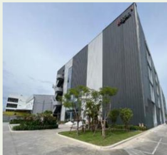
(Thailand – North Bangkok BKK1 Data Center)
